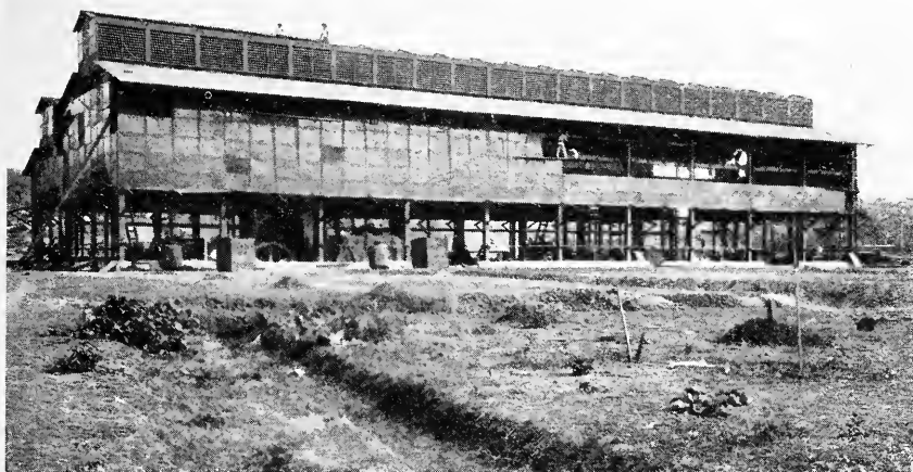
THE PUMPING STATION AT PLATO
